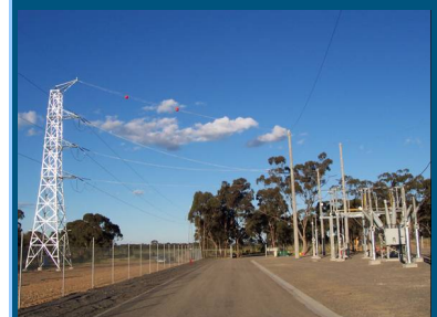
PNS also designed and constructed the new lattice Tower Tee Off
